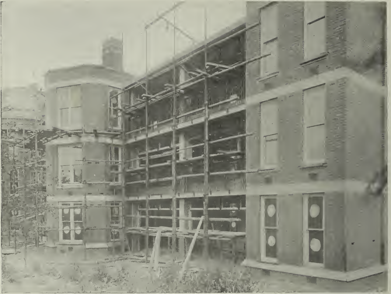
VI.—View of part of the new building of the Children's Hospital (not yet opened) to show the arrangement for open-air treatment for all the children and the provision of shelter while dressing is going on.
